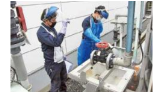
Wastewater neutralization treatment
